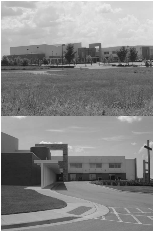
Figure 1. Westside Family Church, Kansas City. Source: authors.
